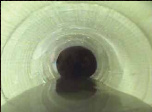
AFTER HAMMERHEAD POINT REPAIR
