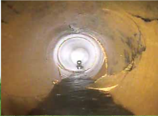
BEFORE HAMMERHEAD® POINT REPAIR
